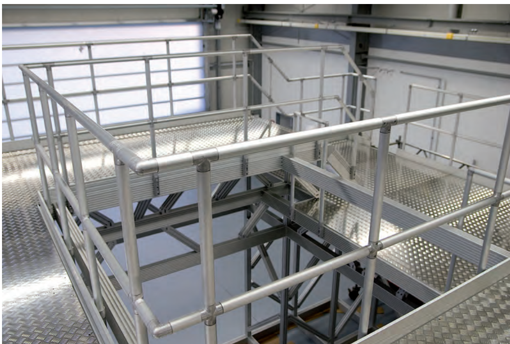
Working platform with ITAS railing
